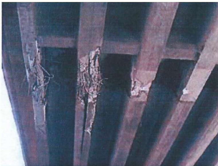
Illustration 12 - Multiple beams damaged by an impact
