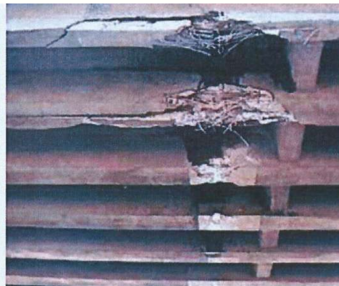
Illustration 12 - Multiple beams damaged by an impact
