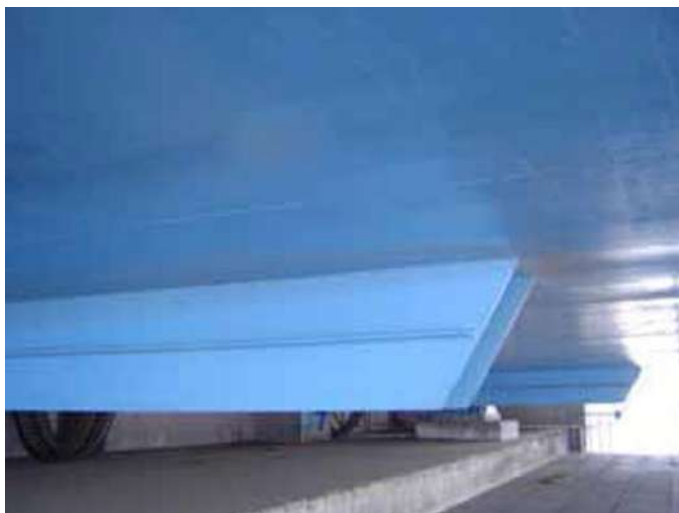
Inspection after 8 years
