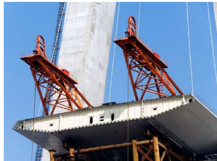
Assembly of sections
