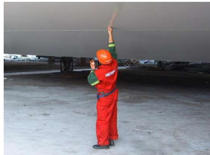
Quality control of coatings
